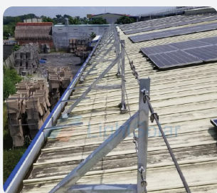
Hàng rào an toàn Safety barriers/fencing
