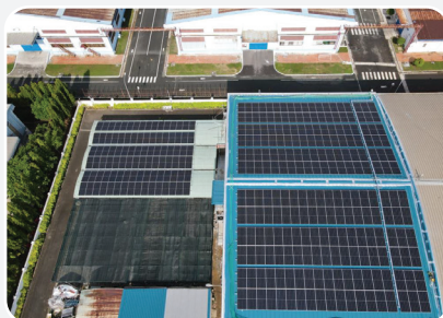
NM QRSF - Vũng Tàu QRSF Factory - Vung Tau Công suất/Capacity: 750MWp
